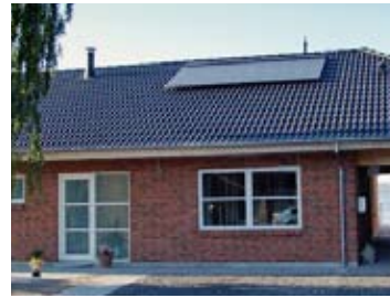
60 tube installation for domestic hot water and space heating
