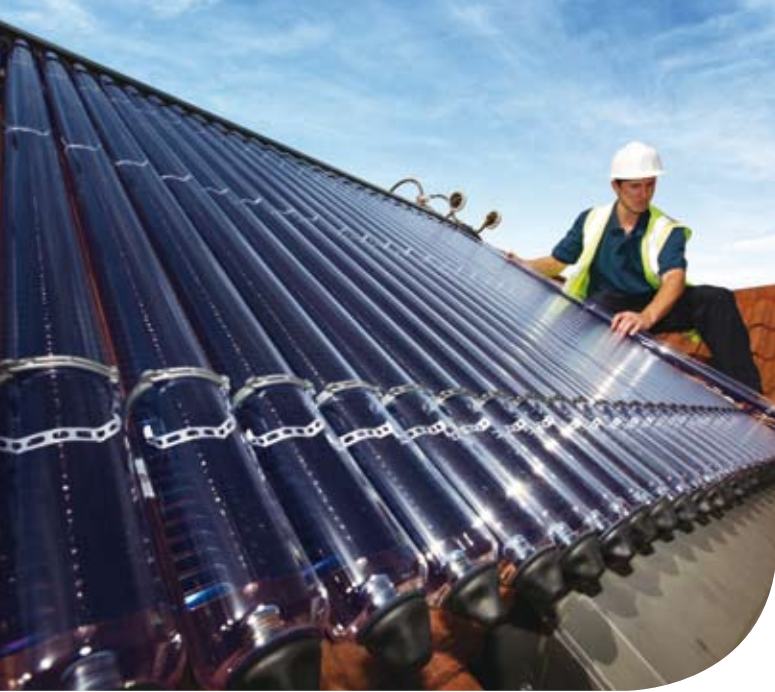
60 tube installation for domestic hot water and space heating
