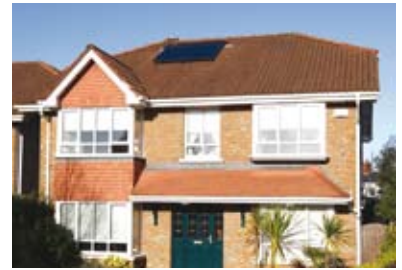
30 tube installation for domestic hot water
